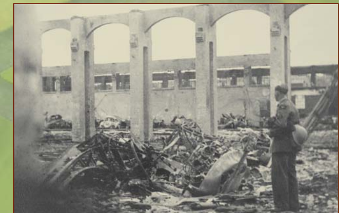
An airman reflects on the wreckage of a hangar after the 18th August attack.
